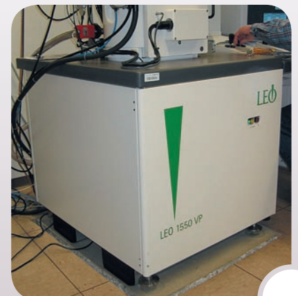
▲ Installation completed, Duo 73 is nearly "invisible" under the SEM
